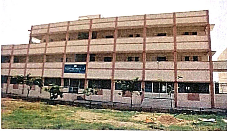
Nine Class rooms-RUSA-PART A-New Construction
