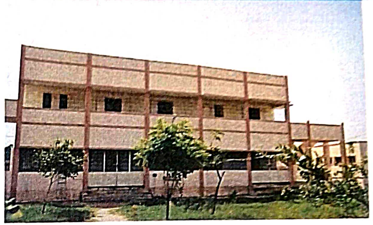
Two Class rooms -RUSA-PART B-Renovation/Up
